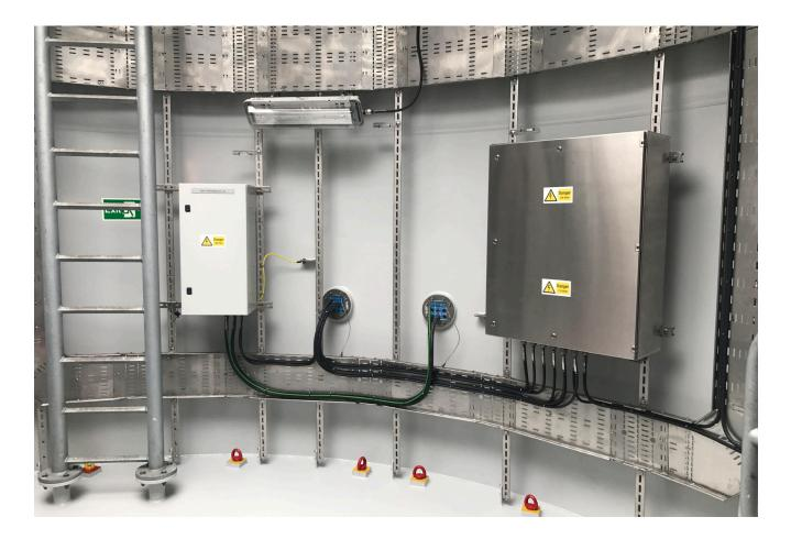
The Fathom LVDB is installed deep within the Wind Turbine Transition Piece, its key role to provide power and light to the Tower area above.
